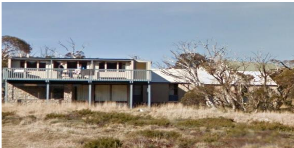
Figure 3 | Photograph of existing western elevation of building (Source: Applicant's documentation)
